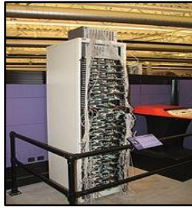
Figure 11: The Google data centre in 1998
