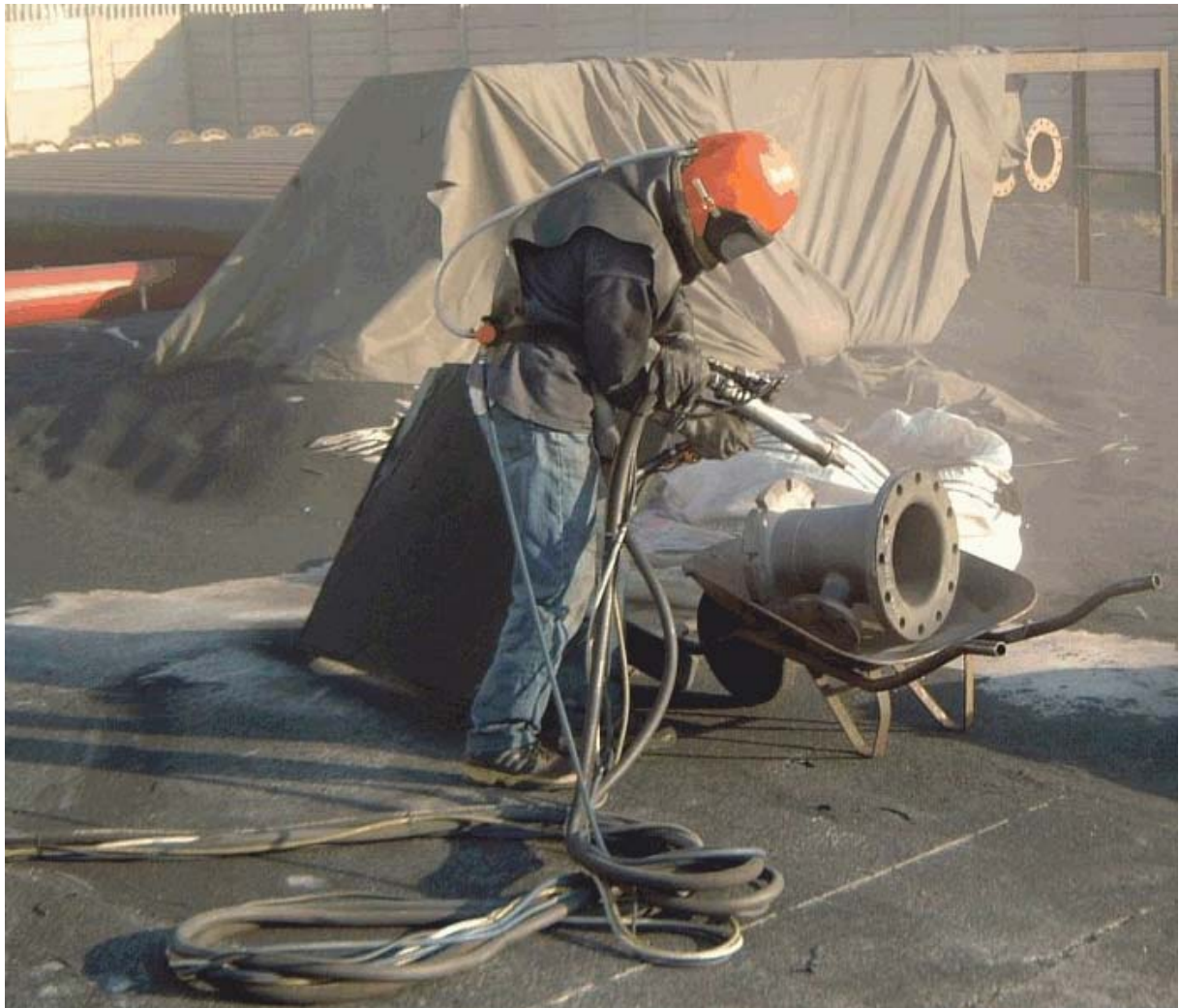
Figure 9: Thermal gun in operation
