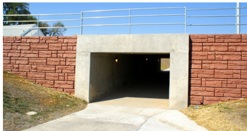
Figure 6: Underground tunnel for pedestrians and bicyclists in Lincoln, NE, USA [22]
